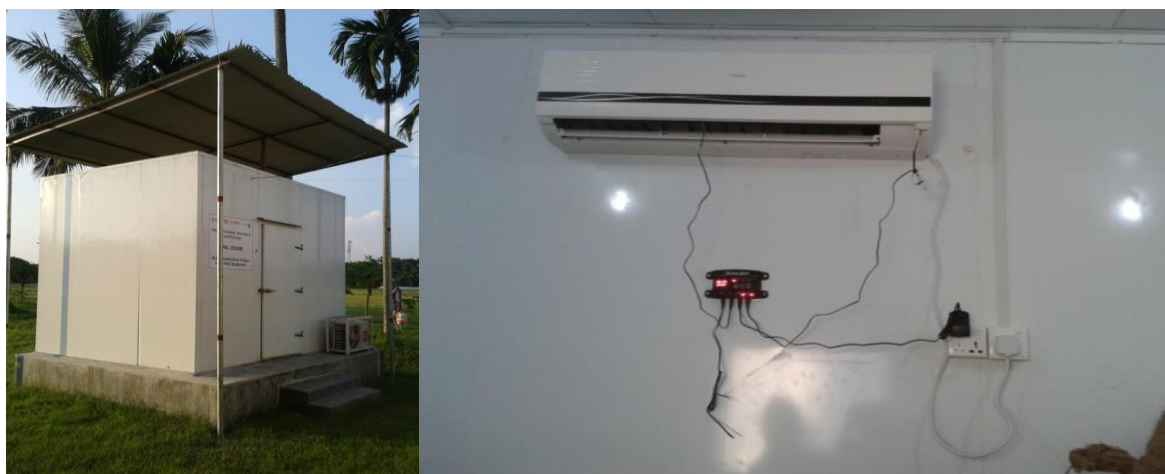
Figure 11. (Upper) CoolBot cold storage, (lower) CoolBot device connected to indoor unit of a room air cooler (Image Source: USAID Horticulture Project, RARS, BARI, Jessore)
